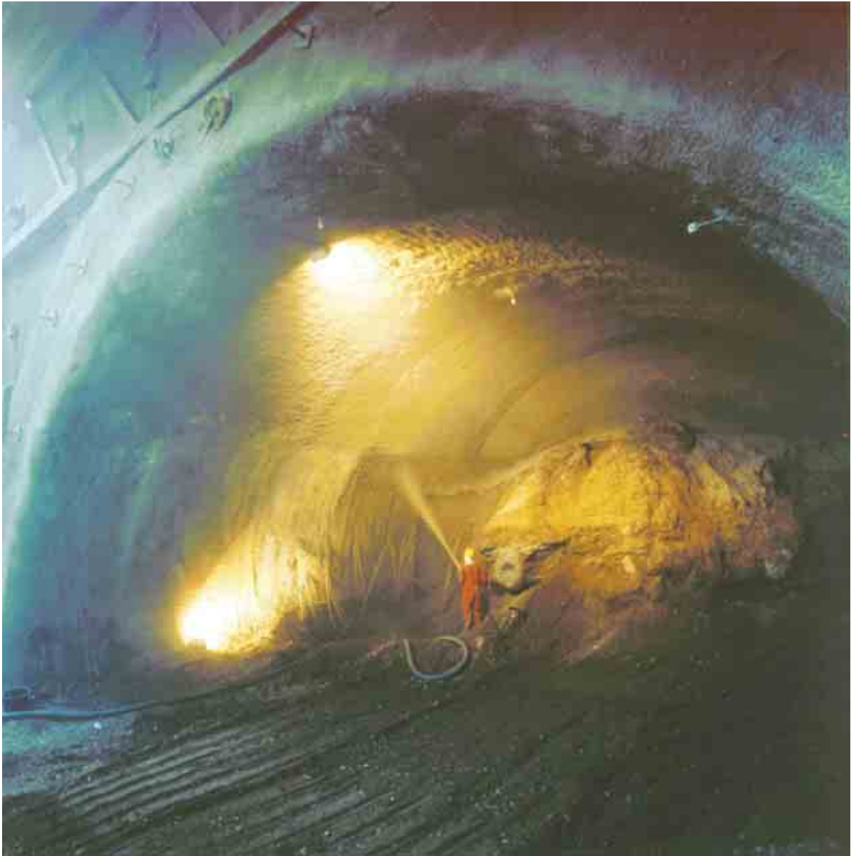
Fig. 7.9: View of the temporary tunnel face
