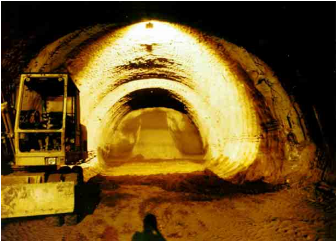
Fig. 7.12: Tunnel face with support core and niche for the construction of the jet grouting columns
