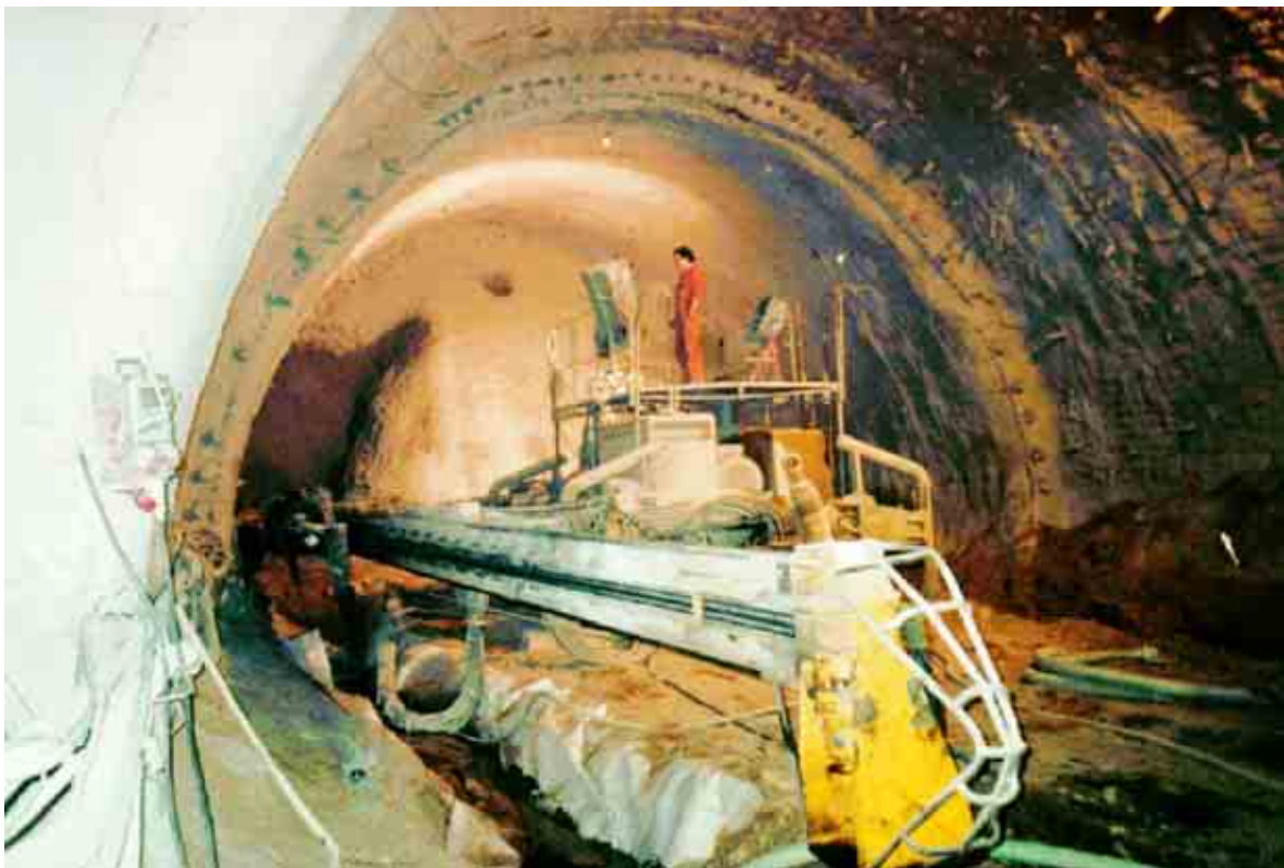
Fig. 7.13: Jet grout drill carriage in operation
