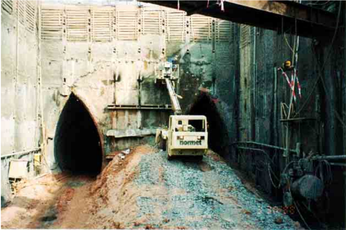
Fig. 5.29: Limburg Tunnel, start of underground excavation at the northern portal
