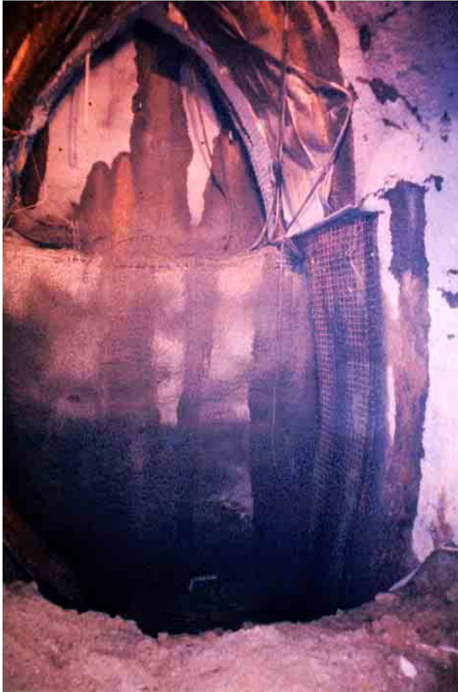
Fig. 5.65: Tunnel face support of the sidewall adit, crown and bench
