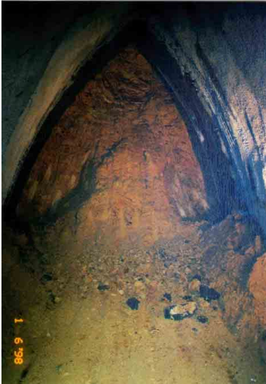
Fig. 5.33: Excavation of the crown of the sidewall adit
