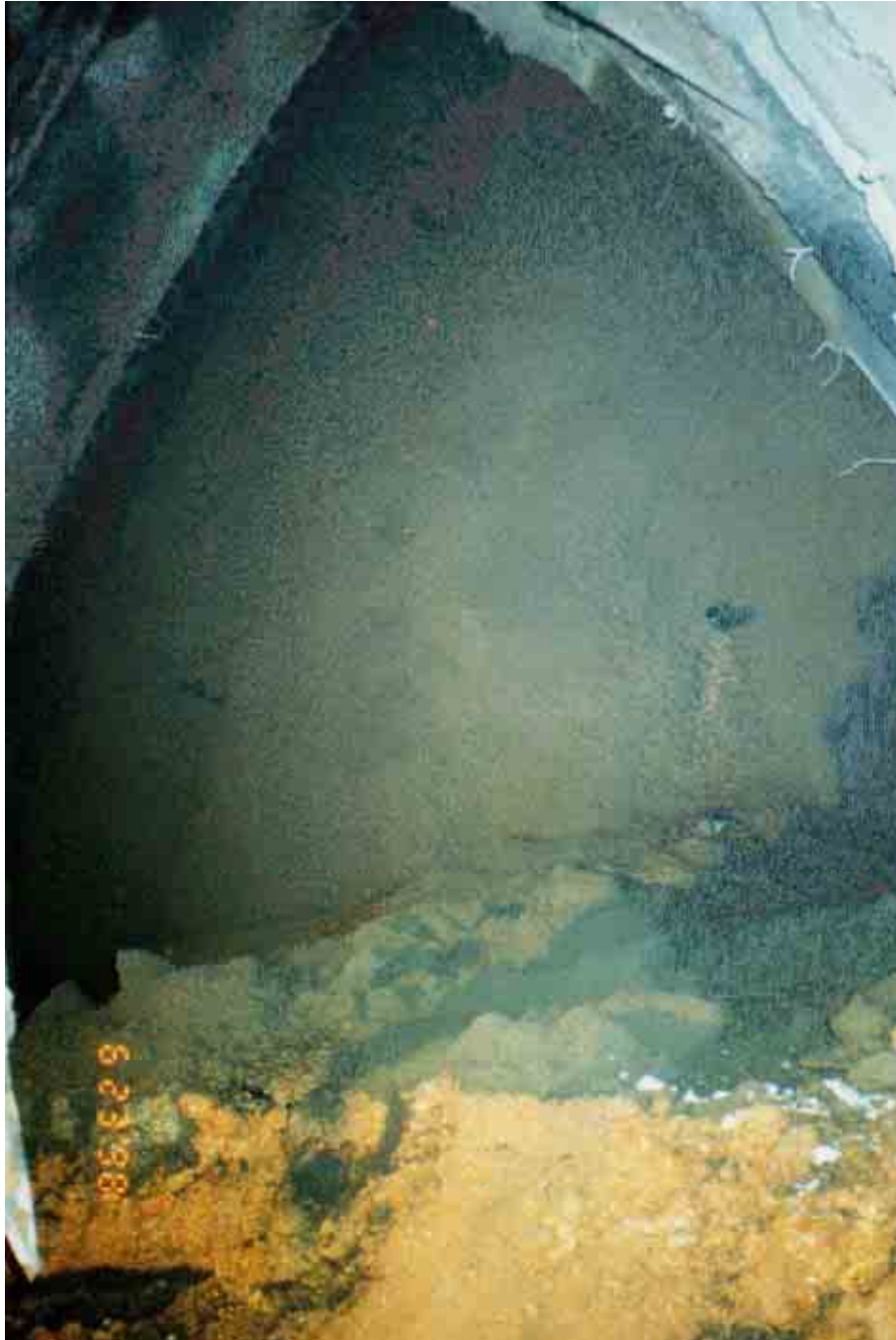
Fig. 5.64: Tunnel face support of the sidewall adit, crown
