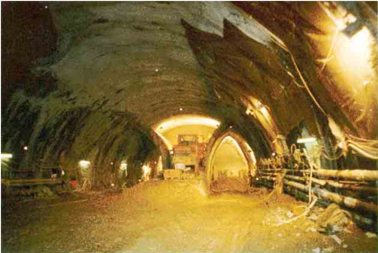
Fig. 5.67: Excavation of the core
