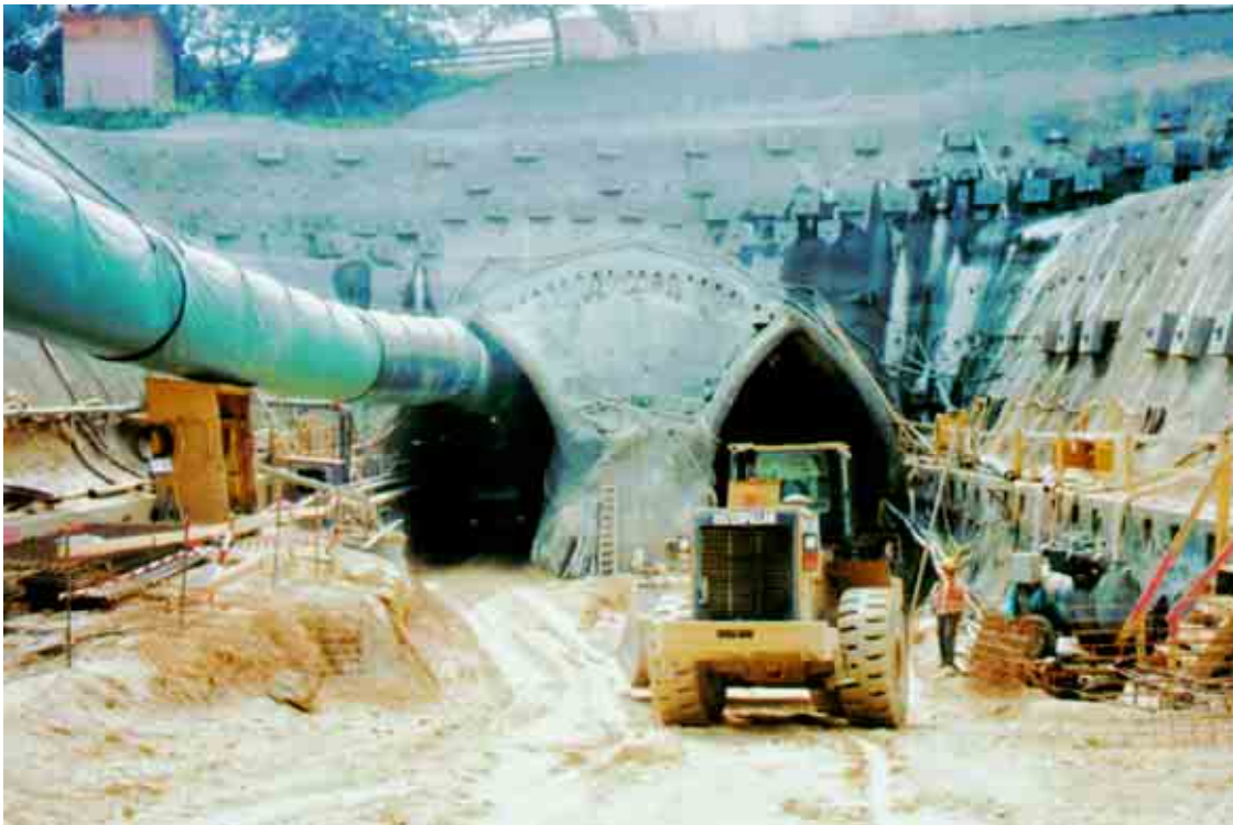
Fig. 5.47: Niedernhausen Tunnel, starting wall of the northern heading
