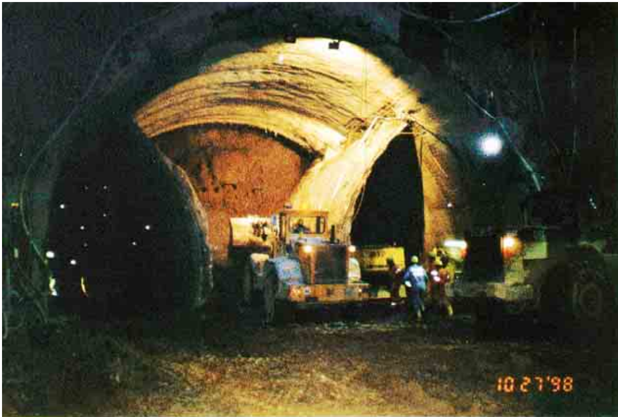
Fig. 5.38: Excavation north, core excavation
