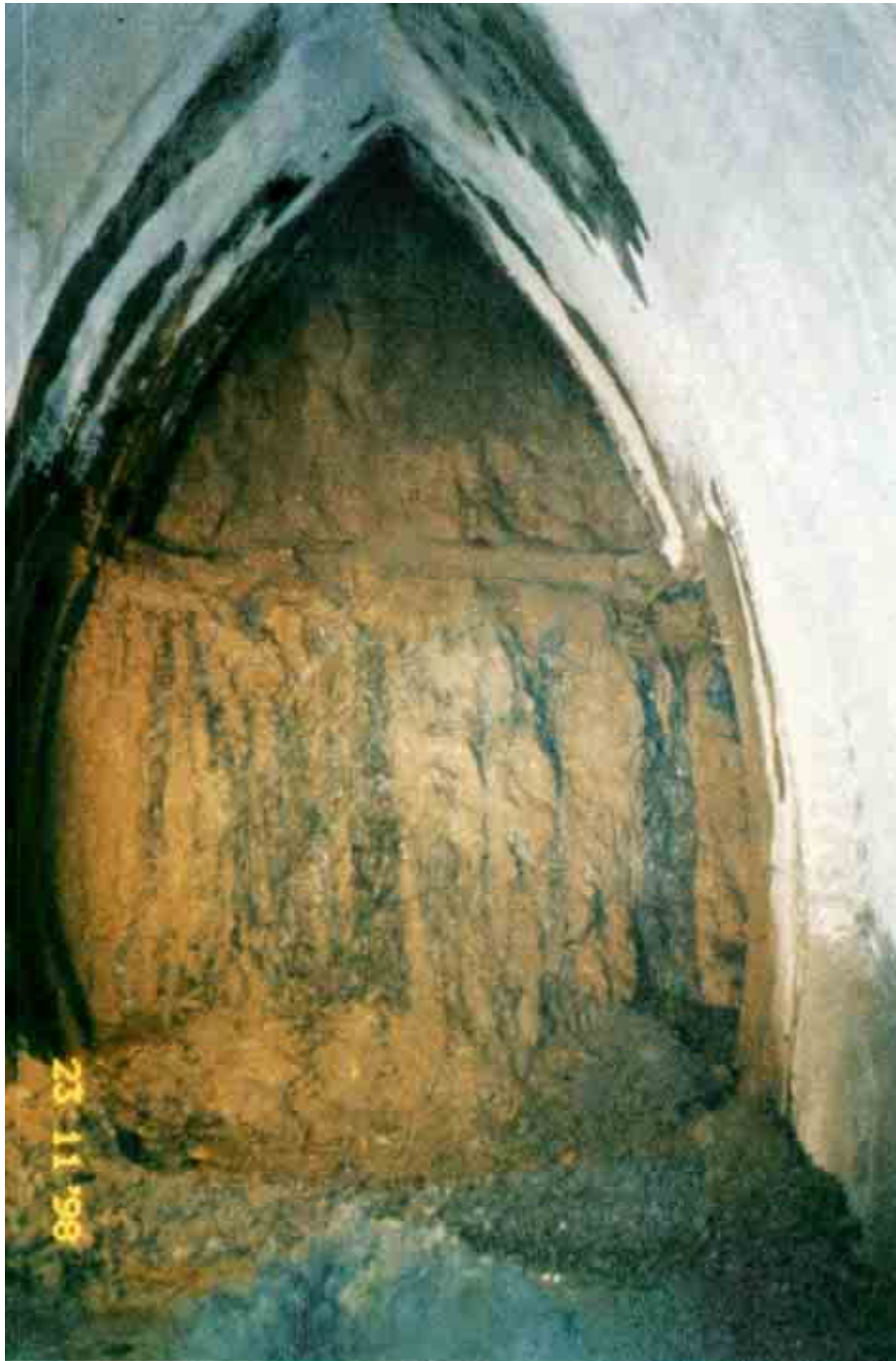
Fig. 5.34: Excavation of the bench of the sidewall adit
