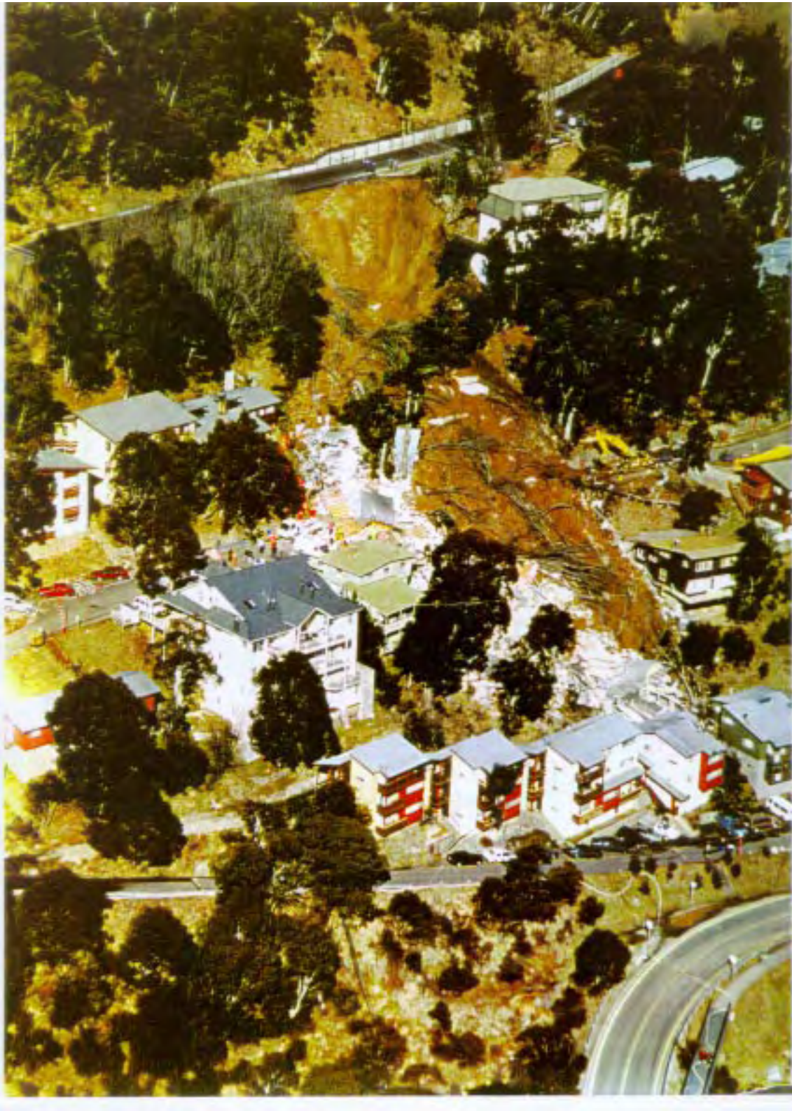
Figure 2. Aerial view of the landslide.
